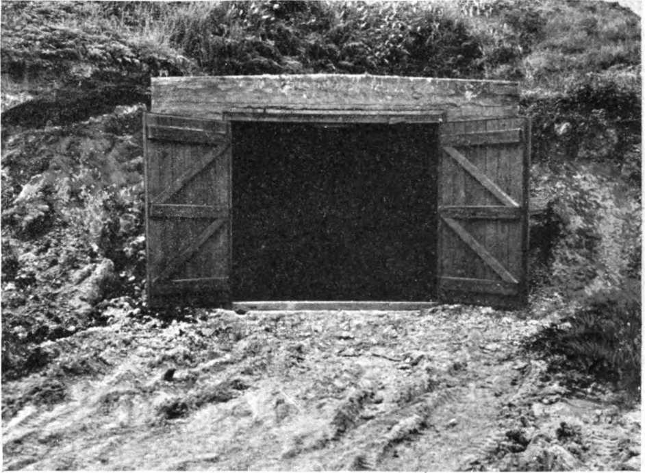
Figure 143. Bomb juze storage constructed in a sidehill.
